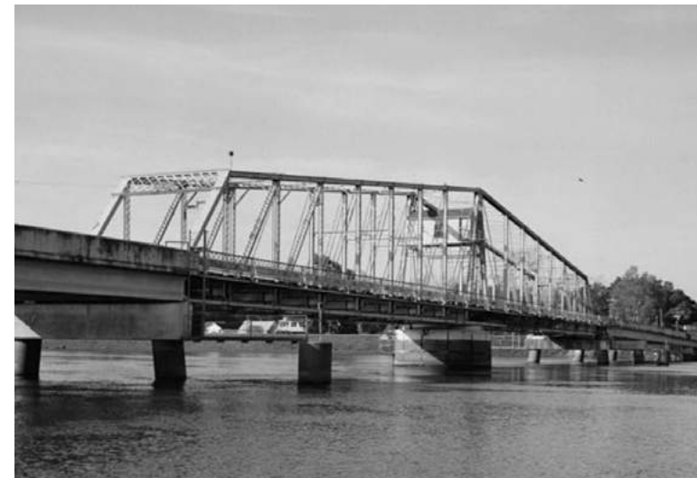
23. ENDOM BRIDGE The DeSiard Street Bridge (Endom Bridge) is what remains of one of the fourteen surviving vehicular swing bridges in the State of Louisiana. The original swing span represents the only Pratt type through truss with a sloped top chord in the State of Louisiana. It was financed and built by the City of Monroe and represents an important part of local and regional history for its contribution to the development of the local and regional economy.
