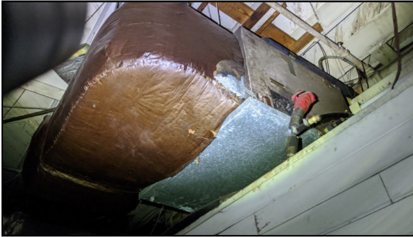
PHOTO 31 Duct insulation in former bottling plant.
