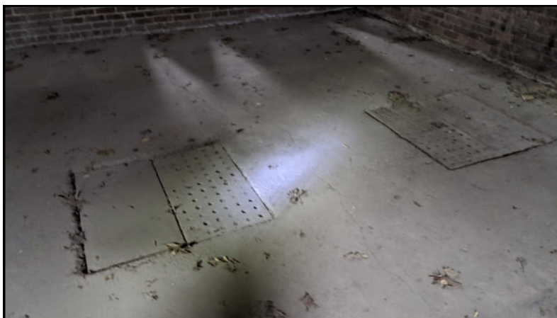
PHOTO 18 Drains in floor of storage area.
