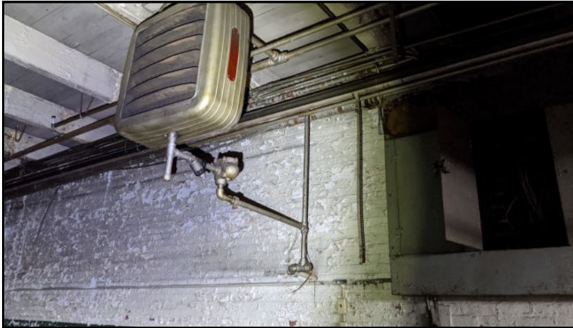
PHOTO 43 Heater unit in production area.
