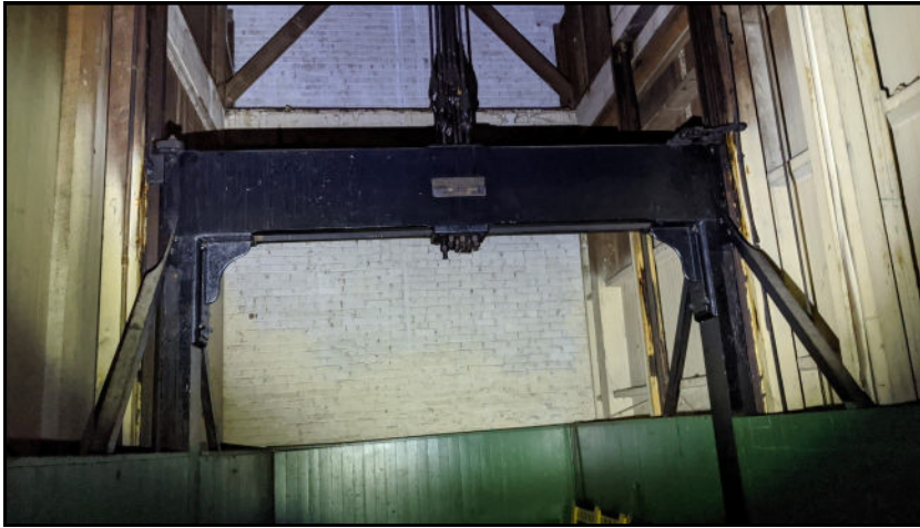
PHOTO 28 Cable operated freight elevator.
