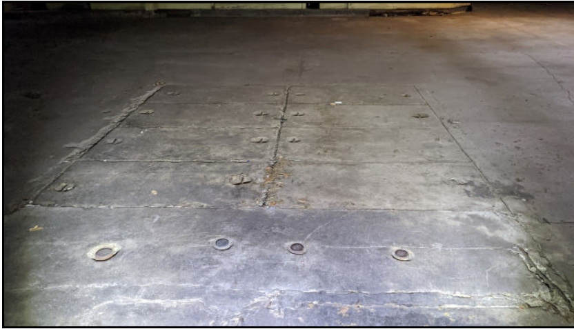
PHOTO 22 Scarring in concrete of stor- age area.
