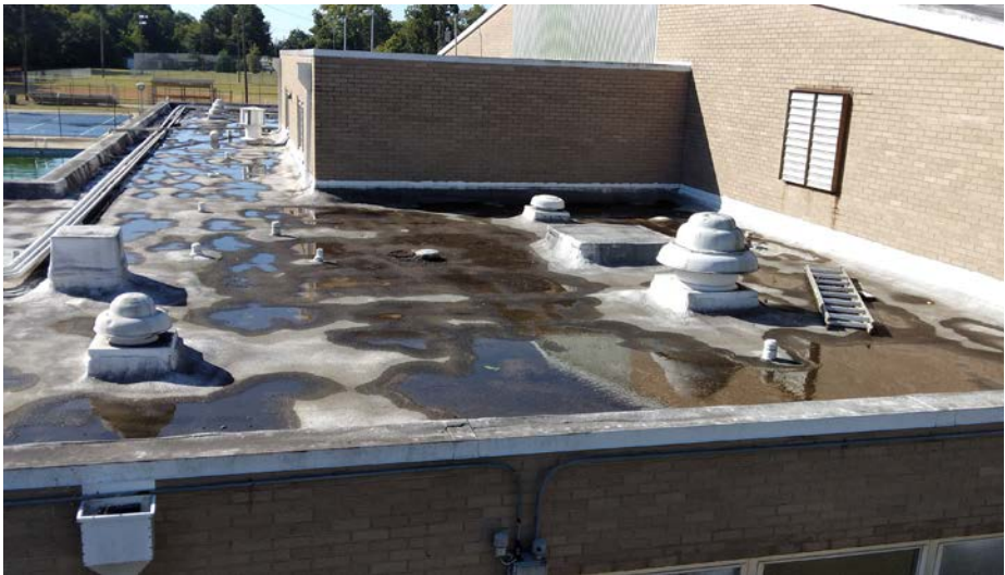
Figure 50: Roof needs to be stripped and replaced
