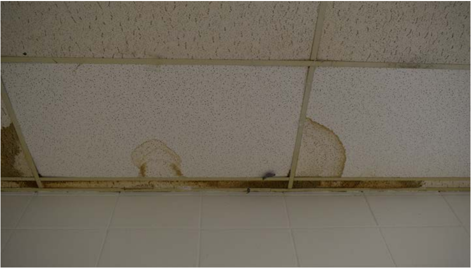
Figure 109: Full ceiling replacement - after roof repair
