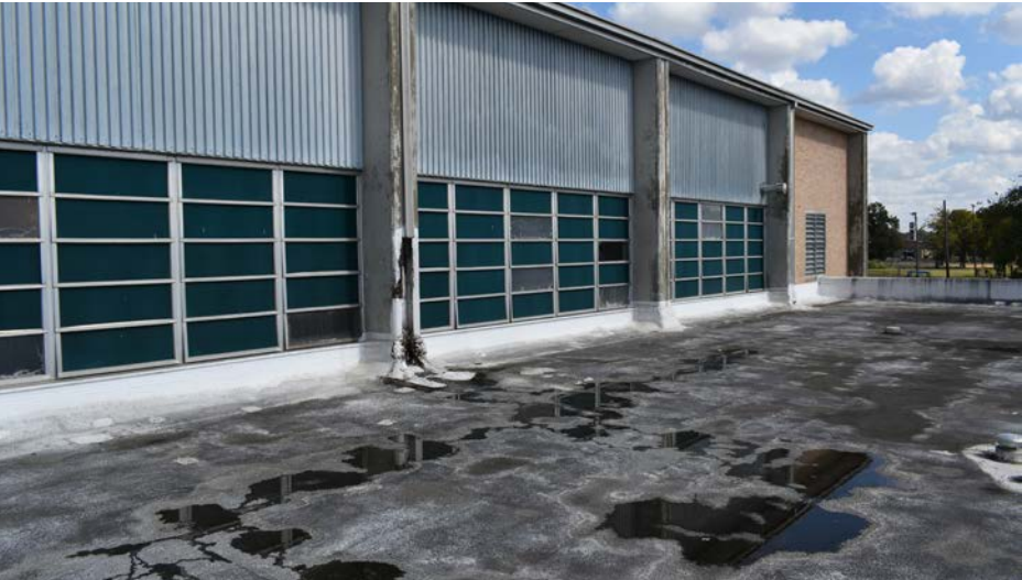
Figure 33: Gym windows are failing and need replacement
