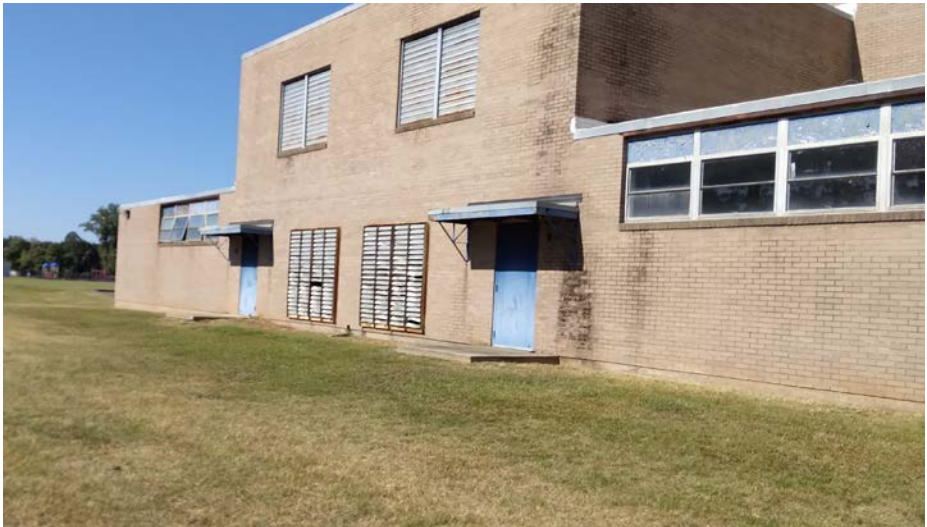
Figure 156: Decaying canopies to be replaced, exterior cleaned
