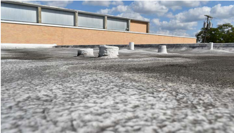
Figure 32: Roof needs to be stripped and resurfaced
