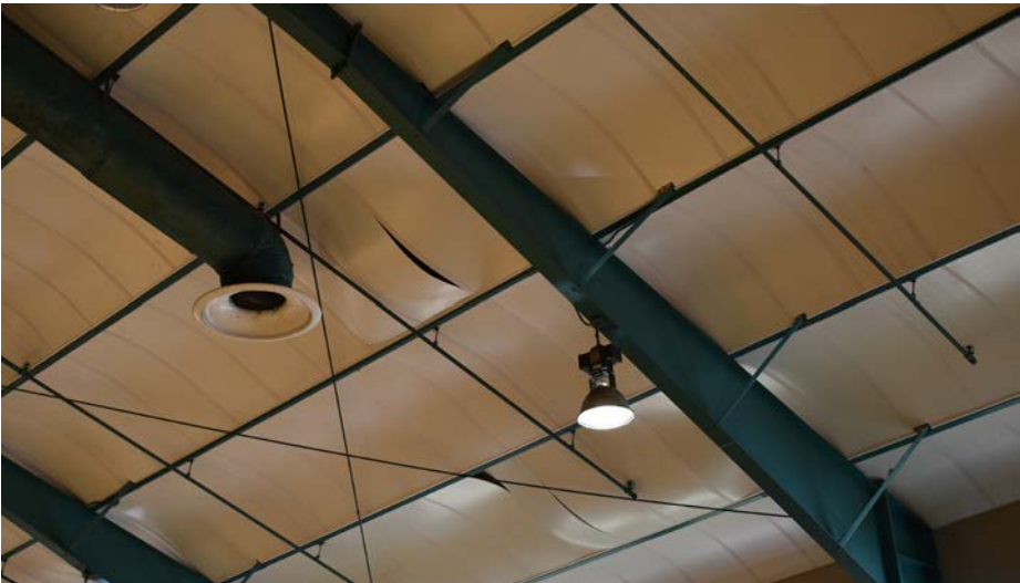
Figure 64: Ceiling panels need replacement - existing leaks
