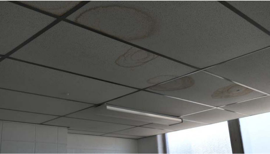
Figure 47: Water damage is visible on ceiling tiles
