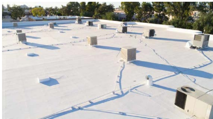
Figure 10: New 20-Year Mod Bit Roof
