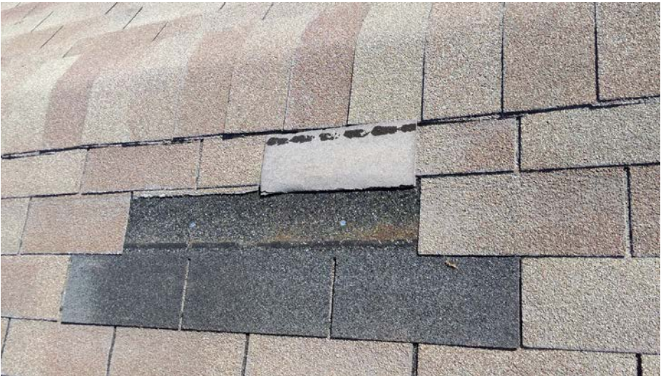
Figure 133: Roof tiles missing and need replacement
