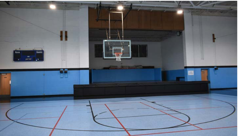
Figure 149: VCT in gym to be replaced with flexible athletic flooring
