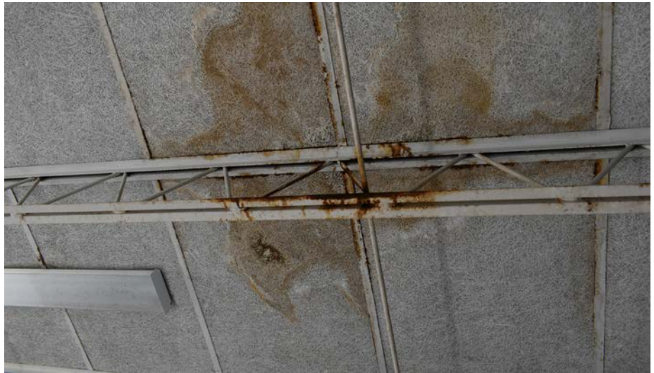
Figure 152: Ceiling damages due to roof leaks
