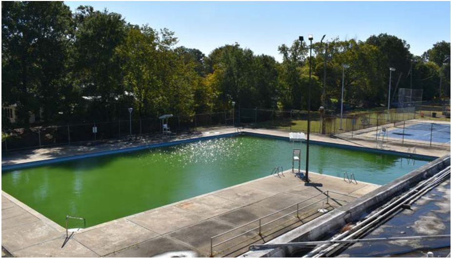
Figure 52: Pool needs to be re-plastered and new decking
