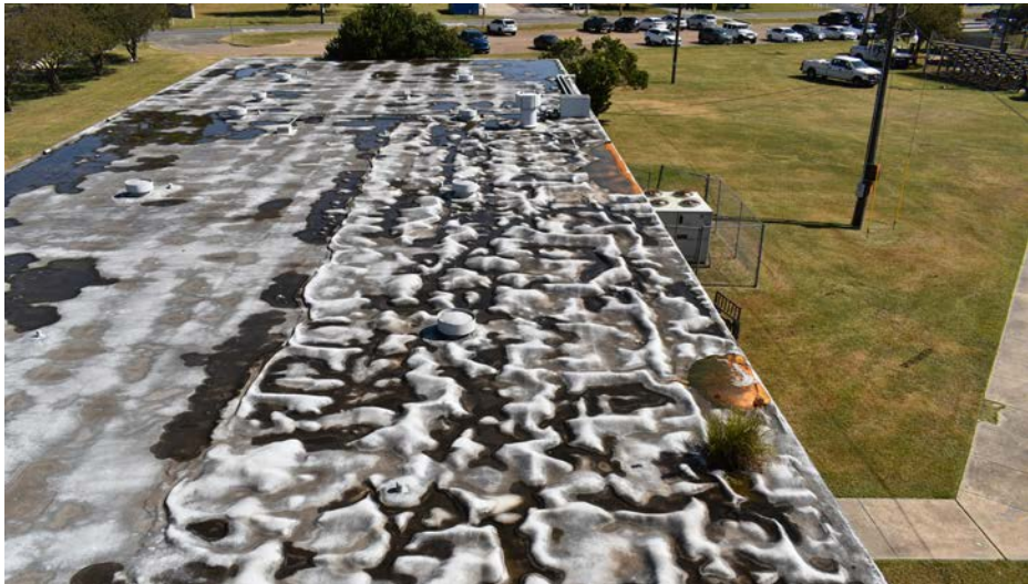
Figure 155: Leaking roof to be removed and replaced
