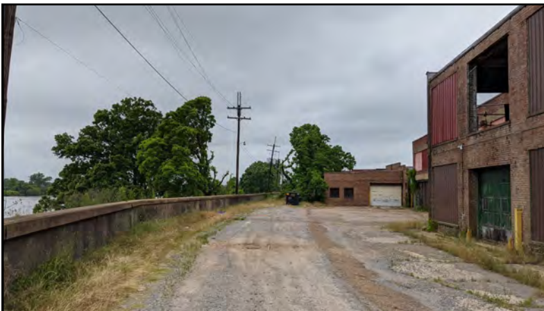
PHOTO 12 West side of the sub- ject property facing north along former rail- way.
