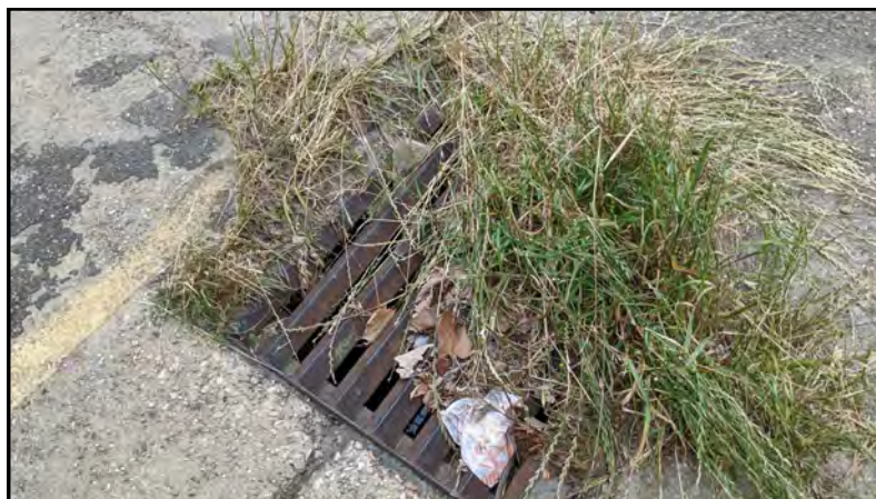
PHOTO 15 Drain on west side of the subject property.
