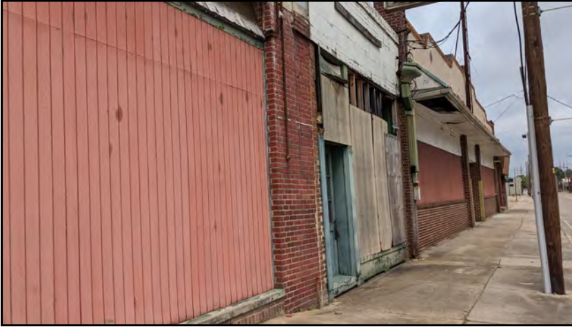
PHOTO 10 Eastern side of the subject property facing to the north.
