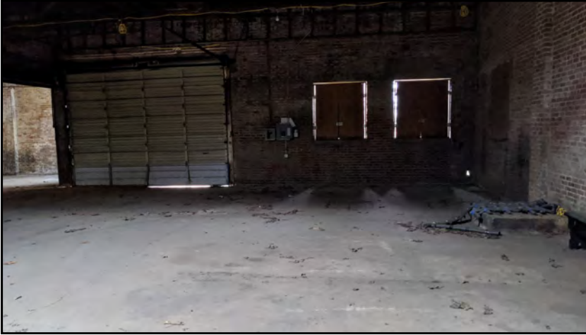
PHOTO 19 Storage area interior.
