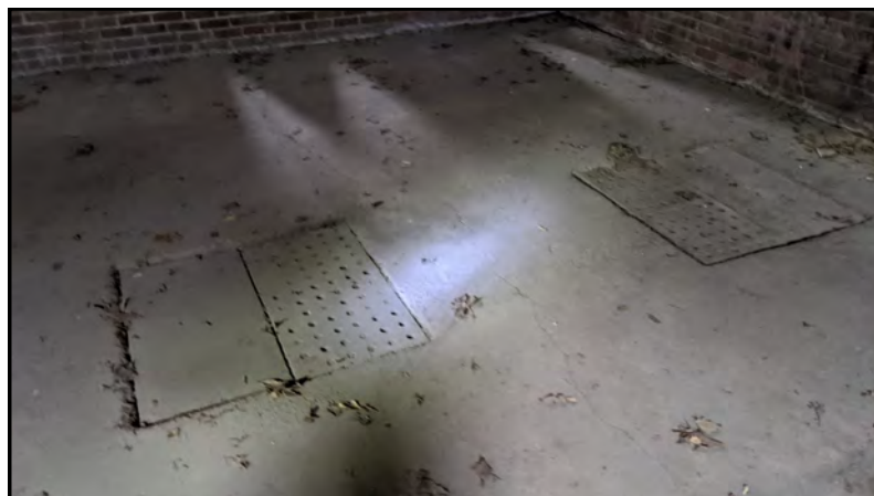
PHOTO 18 Drains in floor of storage area.
