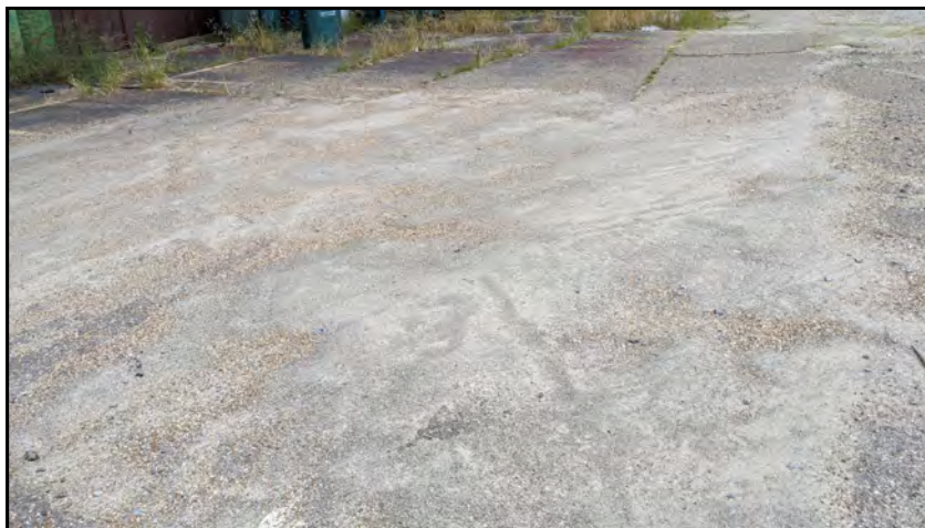
PHOTO 14 Approximately location of former used oil UST pit.
