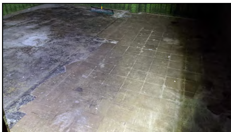
PHOTO 33 Floor tile sample.
