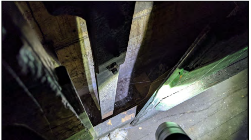
PHOTO 29 Cement flooring beneath elevator.
