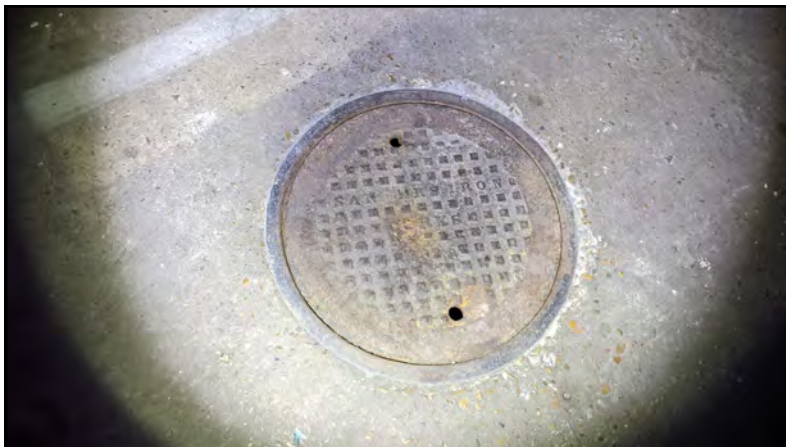
PHOTO 30 Storm drain interior to building.
